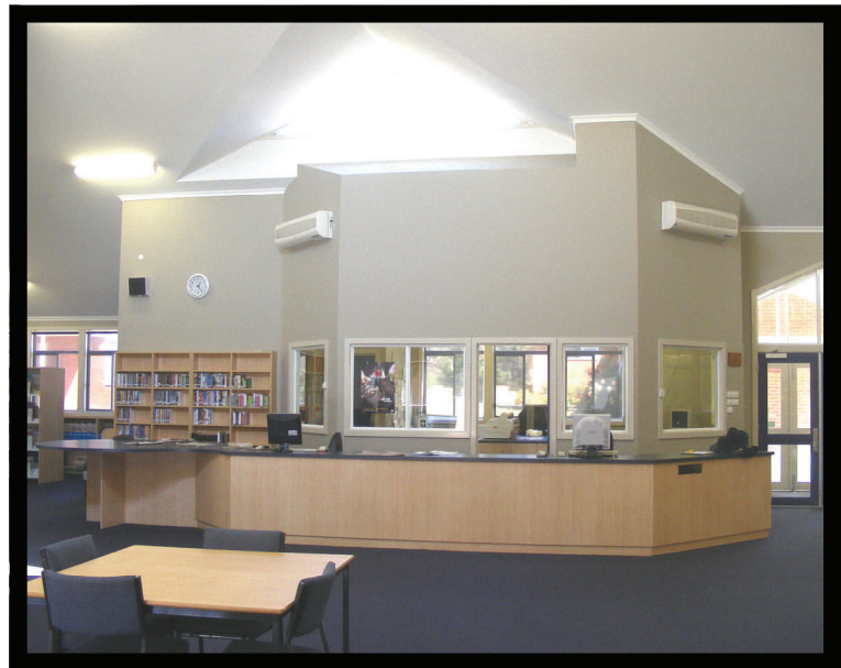
Office, Store, Staff Toilet and Front library desk. All joinery custom made to clients specification.
